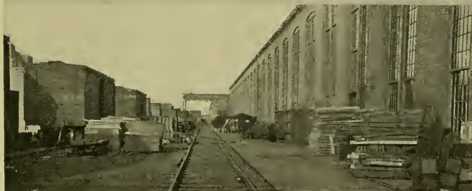
FIG. 72.—SIDE VIEW OF THE PAINT AND FREIGHT CAR SHOPS. PAINT SHOP AT THE RIGHT. FIG. 74.—ONE DAY'S OUTPUT. FIG. 73.—THE FINISHED CAR, READY FOR WEIGHING. FIG. 71.—STORAGE OF MATERIAL ALONG THE NORTH SIDE OF THE CAR SHOP.
